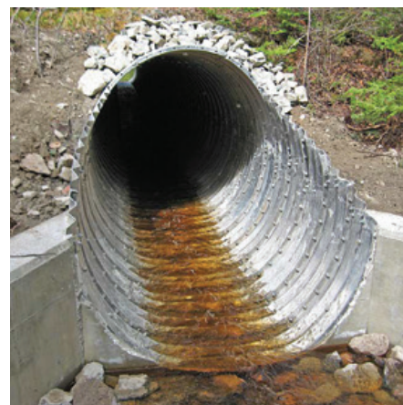
TUNNEL LINER PLATE'S LIGHT WEIGHT MADE IT EASY TO HAND-CARRY SECTIONS TO THIS RESTRICTED ACCESS LOCATION IN TERRA NOVA NATIONAL PARK
