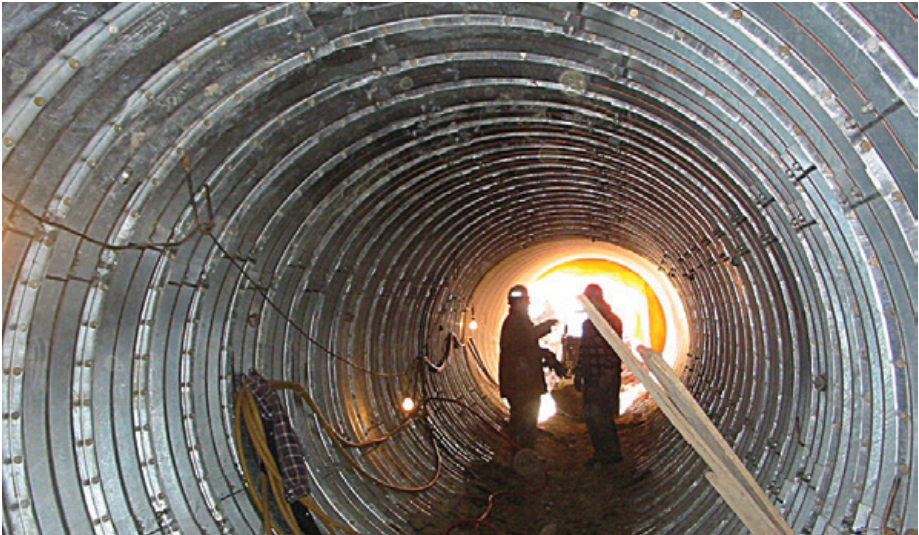
TUNNEL LINER PLATE DELIVERS MAXIMUM STRENGTH WITH MINIMUM WEIGHT
