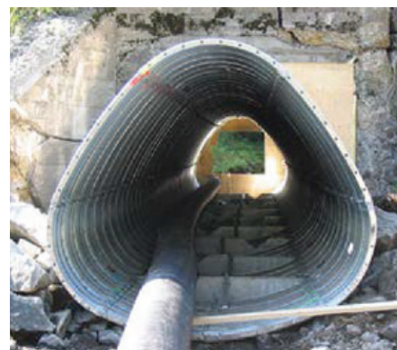
TUNNEL LINER PLATE EARLY INSTALLATION
