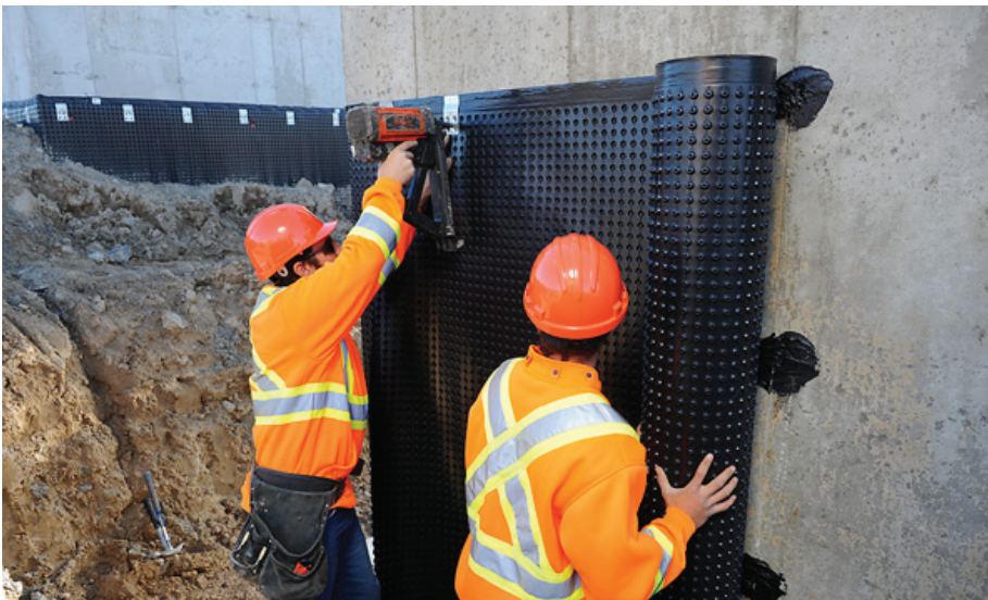
PLATON INSTALLATION - FOUNDATION WALLS
