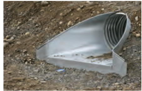
CSP END SECTION WITH OPTIONAL TOE PLATE EXTENSION
