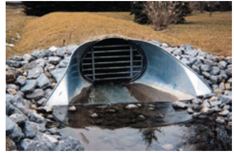
CSP END SECTION WITH FUNCTIONAL GRATE
