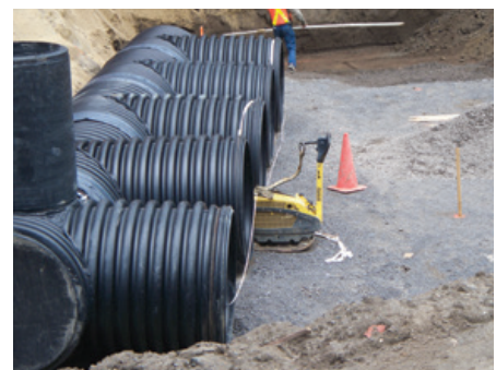
PREPARING THE SOIL FOR HDPE PIPE INSTALLATION
