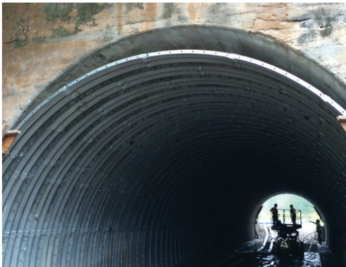
TUNNEL LINER PLATE - TUNNEL RELINE
