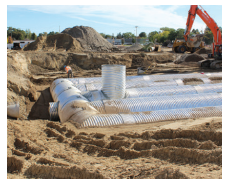
STORMWATER DETENTION SYSTEM
