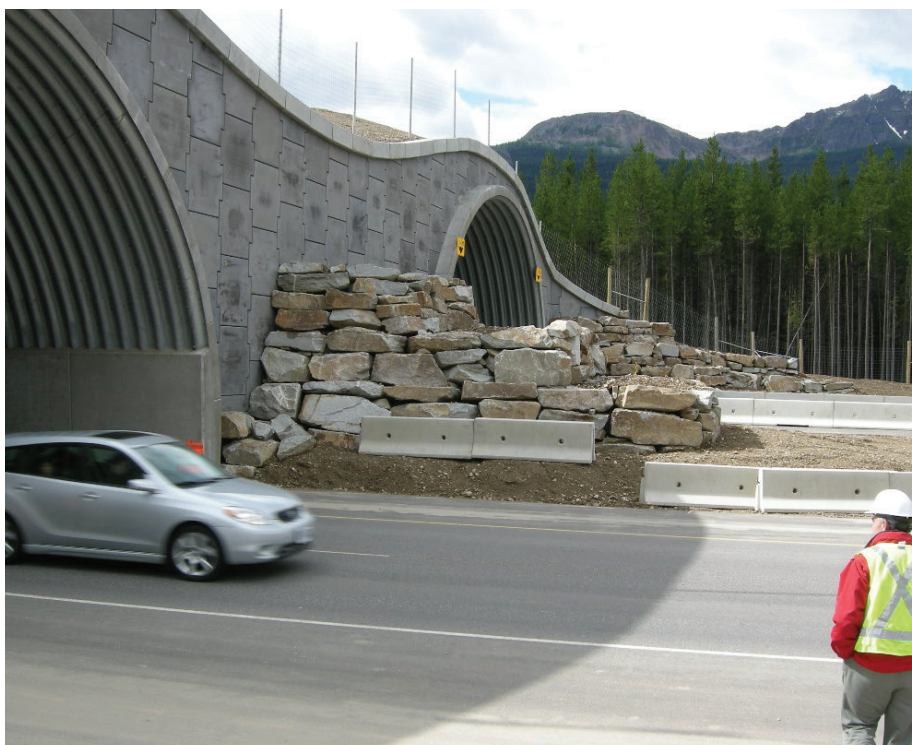
STRUCTURAL PLATE - GRADE SEPARATION
