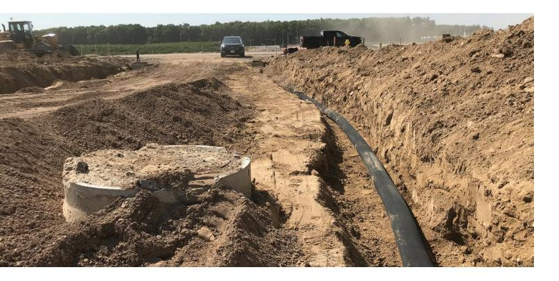
Big O's High Density Polyethylene (HDPE) construction combines strength and durability in a lightweight product. **Meeting ASTM F667** and **AASHTO M252, it is rated to HS-25 Highway Traffic Loads when installed with a minimum 300mm (12in) height of cover.**
