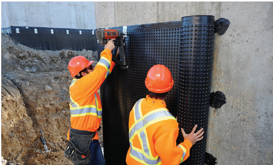
PLATON INSTALLATION - FOUNDATION WALLS
