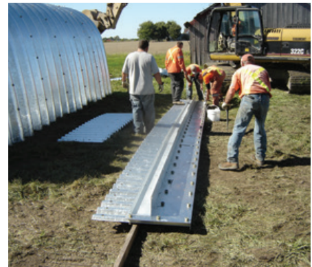
BOX CULVERT WITH STEEL FOOTINGS
