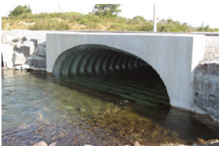
CAST-IN-PLACE CONCRETE HEADWALLS
