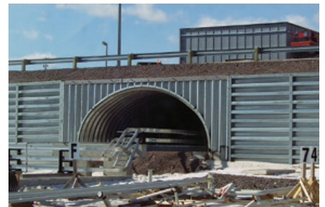
BRIDGE-PLATE HEADWALL AND BIN-WALL WINGWALLS
