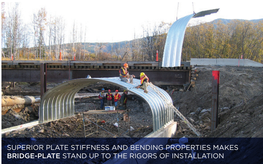
CURVED BRIDGE-PLATE INSTALLATION
