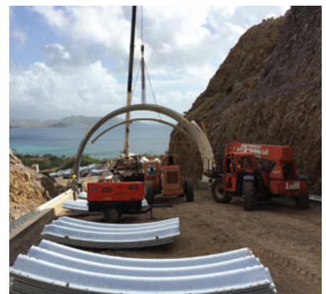
ST. KITTS - COMPONENTS ARE SHIPPED IN NESTED BUNDLES FOR ECONOMICAL TRANSPORTATION
