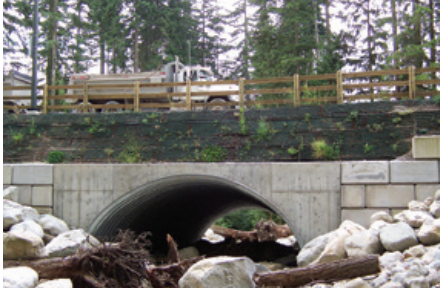
CAST-IN-PLACE HEADWALL WITH SEGMENTAL BLOCK RETAINING WINGWALLS
