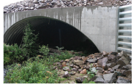
CAST-IN-PLACE CONCRETE HEADWALLS WITH ARMTEC BIN-WALLS
