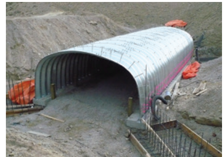
BOX CULVERT WITH PRECAST FOOTINGS
