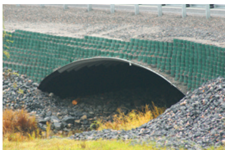
GEOCELL MSE RETAINING WALLS
