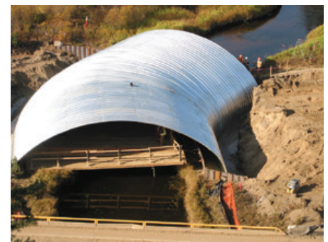
CURVED BRIDGE-PLATE INSTALLATION
