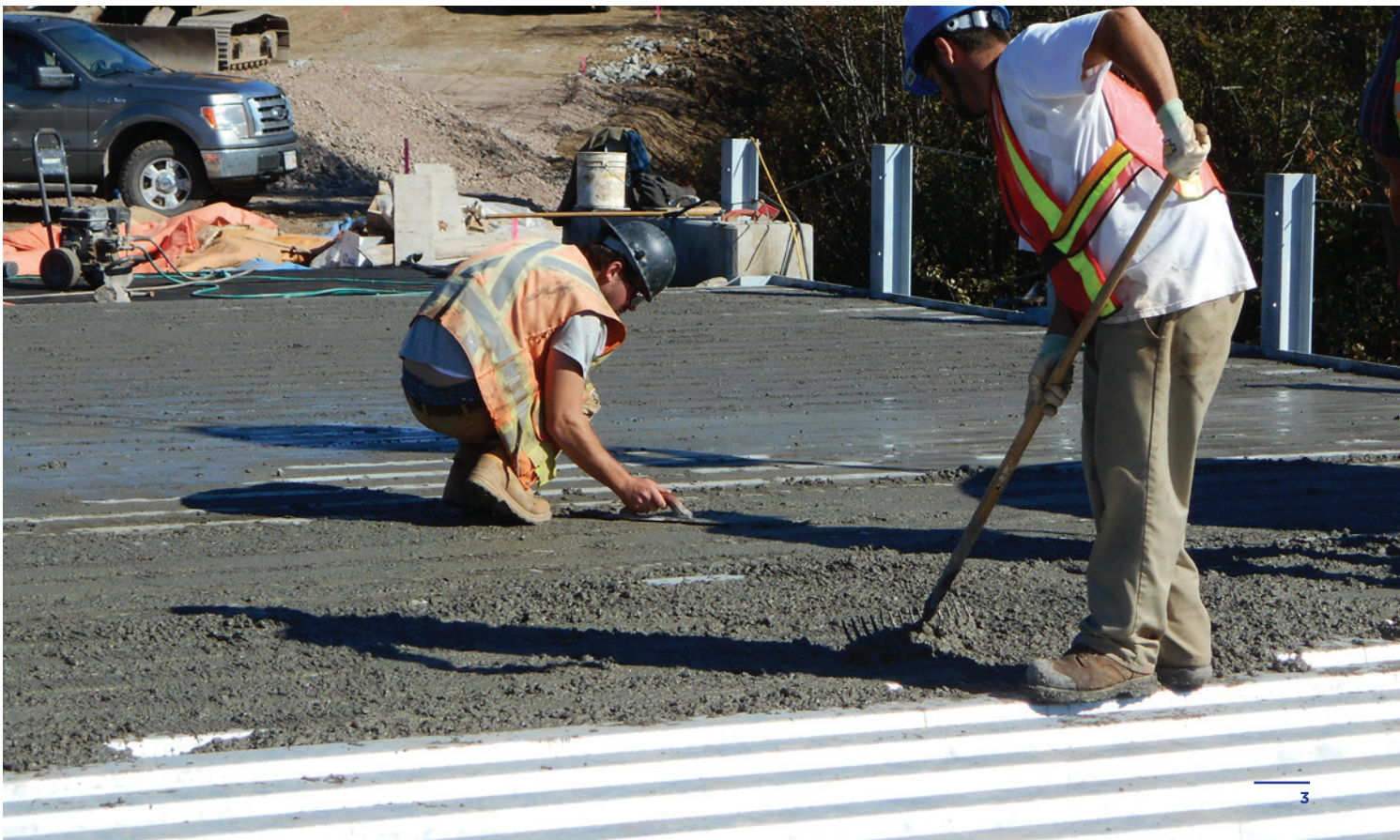
FILLING CORRUGATIONS WITH CONCRETE
