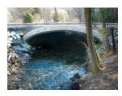
Pre-assembled and pre-engineered open-bottom corrugated steel arch
