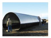
Unique copolymer coating system for structural corrugated steel bridges
