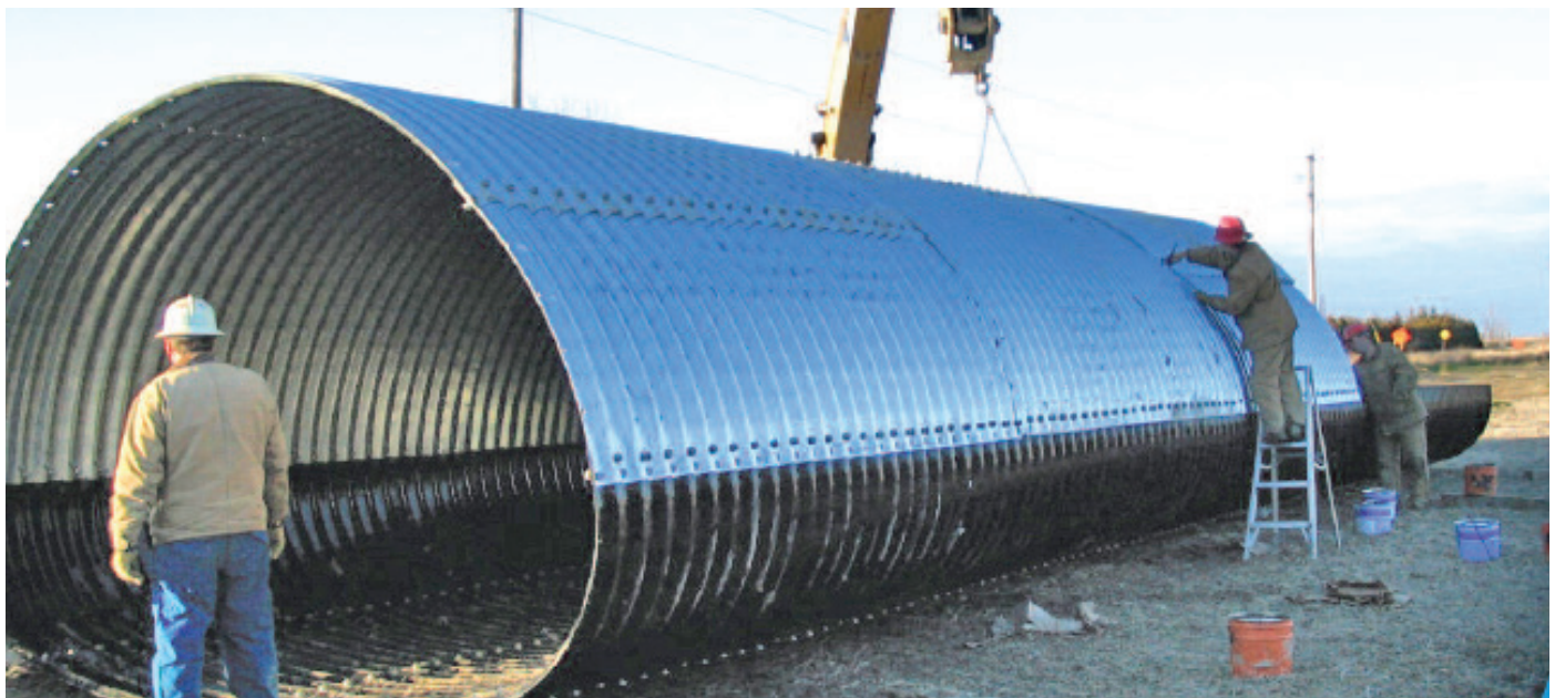
FIRST POLYMER COATED STRUCTURAL PLATE SUPPLIED TO REGIONAL MUNICIPALITY OF CHATHAM-KENT, ON - MULTI-PLATE PIPE-ARCH WITH INVERT PLATES HOT-DIP GALVANIZED COATED WITH POLYMER, AND SIDE AND CROWN PLATES
