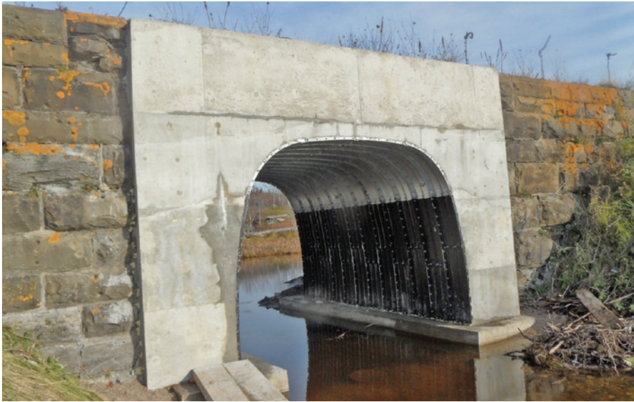
ABOVE AND RIGHT: RAILWAY BRIDGE REHABILITATION - CAPE BRETON NS TUNNEL LINER PLATE WITH STRATA-CAT COATED SIDE PLATES
