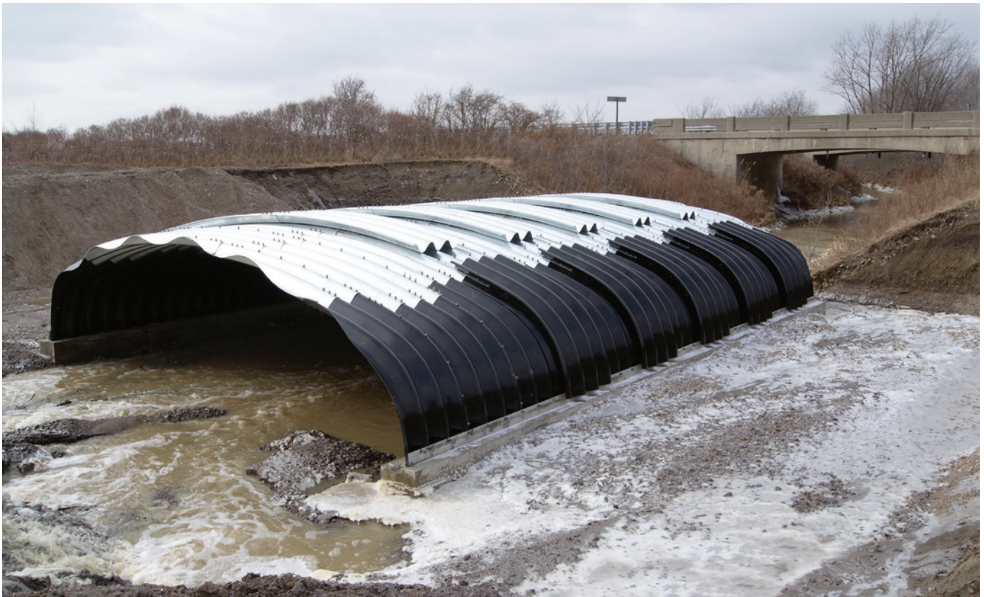
FIRST POLYMER COATED STEEL BOX CULVERT SUPPLIED TO REGIONAL MUNICIPALITY OF CHATHAM-KENT, ON - BRIDGE-PLATE BOX CULVERT WITH SKEWED ENDS, HOT-DIP GALVANIZED CROWN PLATES AND RIBS, AND STRATA-CAT COATED SIDE PLATES AND RIBS
