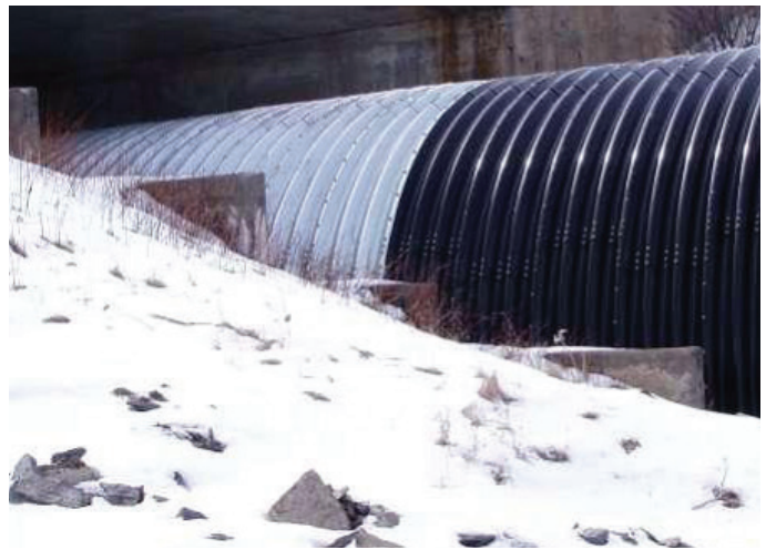
FIRST POLYMER COATED STRUCTURAL PLATE SUPPLIED TO MINISTRY OF TRANSPORTATION OF ONTARIO (MTO), HIGHWAY 401 - BRIDGE-PLATE ARCH WITH POLYMER COATING ON OUTSIDE OF ENDS
