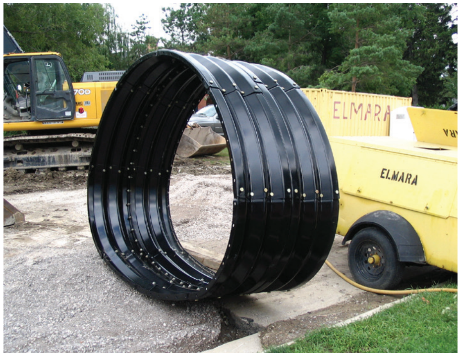
FIRST POLYMER COATED TUNNER LINER PLATE SUPPLIED TO REGIONAL MUNICIPALITY OF CHATHAM-KENT, ON - TUNNEL LINER PLATE PIPE-ARCH RELINE PROJECT WITH STRATA-CAT COATING
