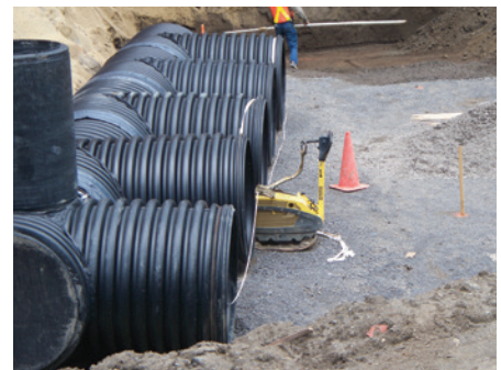
PREPARING THE SOIL FOR HDPE PIPE INSTALLATION
