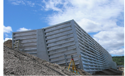
BATTER BINWALL BETTER ACCOMMODATES MINOR GROUND MOVEMENT
