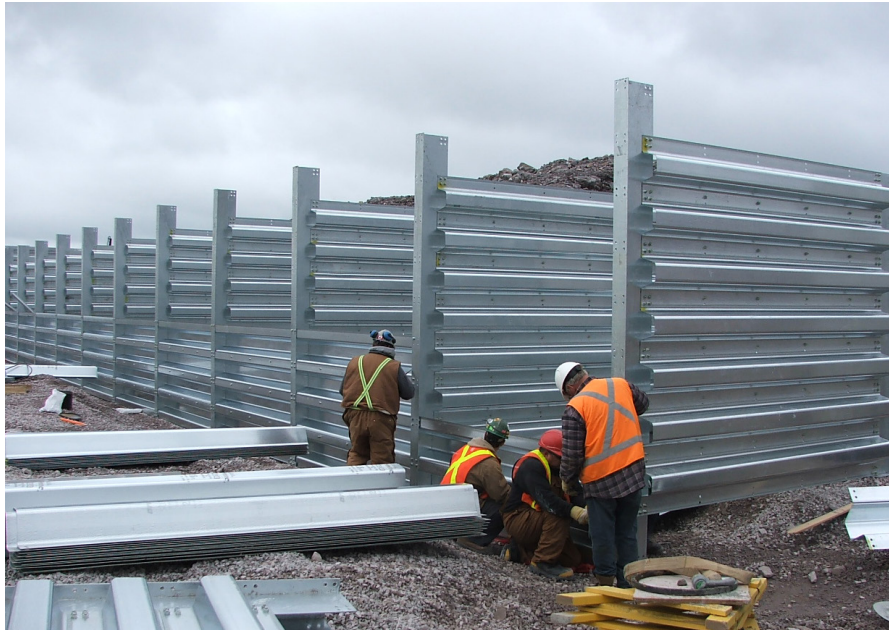
BINWALL ASSEMBLY IS QUICK AND EASY
