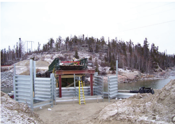
BIN WALL COMPONENTS ARE EASILY BOLTED TOGETHER TO FORM A VARIETY OF CONFIGURATIONS
