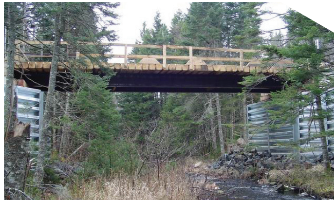
AN ECONOMICAL ALTERNATIVE TO CONCRETE BRIDGE ABUTMENTS
