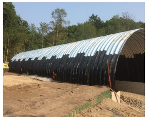
Located beneath the City's bicycle path, the chambers were installed between the road and the backyards of neighbouring homes. The tight space along the roadway had many interfering structures such as Hydro poles, trees, and a drainage ditch on either side. Armtec provided specific drawings to address the complex footprint and accommodate both the existing and proposed structures.
