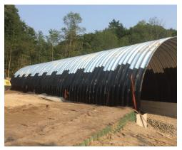
Located beneath the City's bicycle path, the chambers were installed between the road and the backyards of neighbouring homes. The tight space along the roadway had many interfering structures such as Hydro poles, trees, and a drainage ditch on either side. Armtec provided specific drawings to address the complex footprint and accommodate both the existing and proposed structures.
