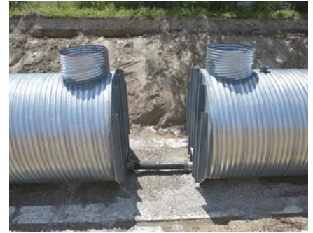
GALVANIZED CSP STORMWATER TANK SYSTEM
