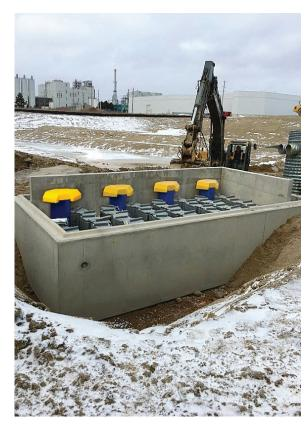
The system is certified by the New Jersey Department of Environmental Protection (NJDEP) and the City of Toronto, to have a removal rate of >80% Total Suspended Solids (TSS). This was critical to the project as the water would eventually flow into the existing storm sewer network.
