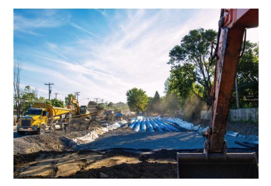
Located beneath the City's bicycle path, the chambers were installed between the road and the backyards of neighbouring homes. The tight space along the roadway had many interfering structures such as Hydro poles, trees, and a drainage ditch on either side. Armtec provided specific drawings to address the complex footprint and accommodate both the existing and proposed structures.
