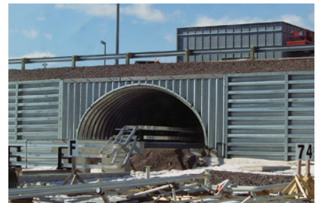
BRIDGE PLATE HEADWALL AND BIN-WALL WINGWALLS
