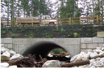
CAST-IN-PLACE HEADWALL WITH SEGMENTAL BLOCK RETAINING WINGWALLS
