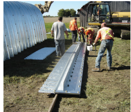
BOX CULVERT WITH STEEL FOOTINGS
