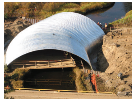
CURVED BRIDGE PLATE INSTALLATION
