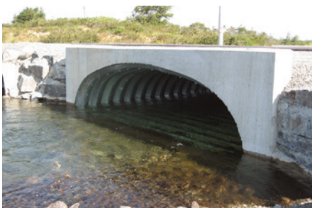
CAST-IN-PLACE CONCRETE HEADWALLS
