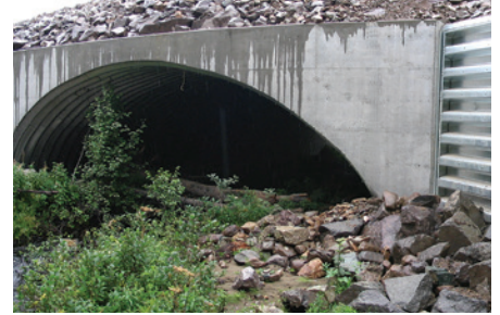
CAST-IN-PLACE CONCRETE HEADWALLS WITH ARMTEC BIN-WALLS
