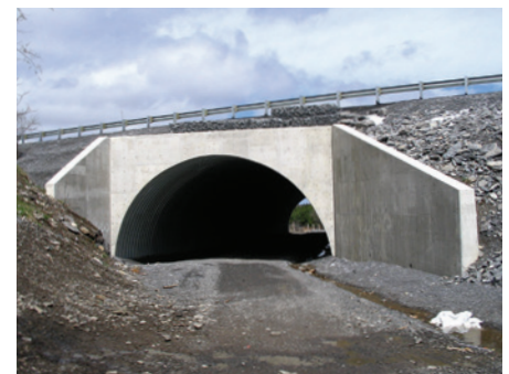
HIGHWAY 401 KINGSTON, ONTARIO - QUICK INSTALLATION REDUCES DISRUPTION TO ROAD USERS
