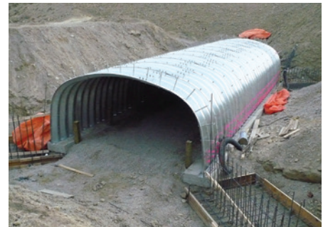
BOX CULVERT WITH PRECAST FOOTINGS
