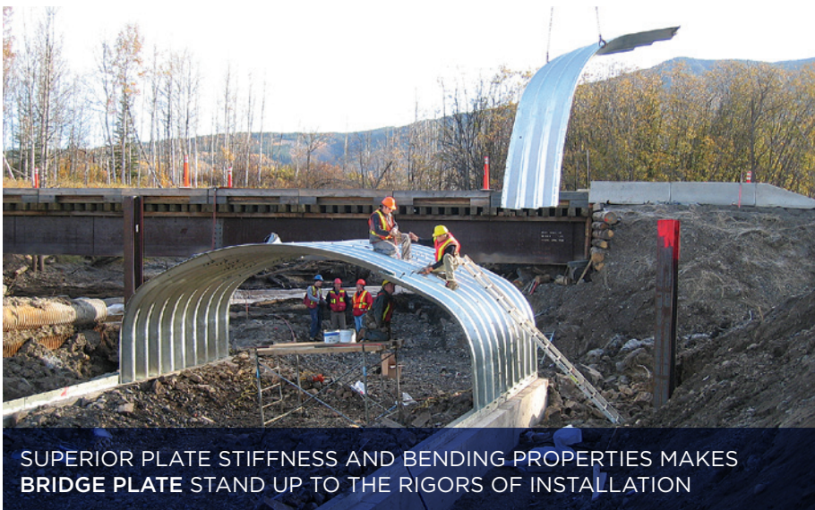
CURVED BRIDGE PLATE INSTALLATION
